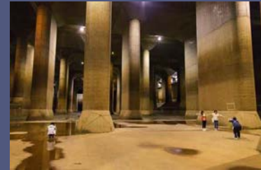
TOKYO STORM WATER DRAINS – WOW!!
